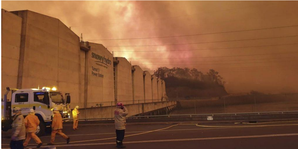
Tumut 3 hydro power plant with 6 turbines (3 pumps) saved by dedicated crew
